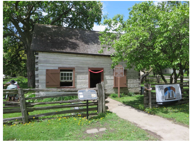
Above: Where the city’s oldest doorway still welcomes visitors, 232 years and counting... Photo: Brent Cunningham
