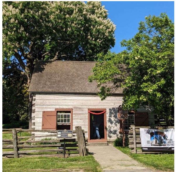
Above: The Scadding Cabin, Doors Open Toronto May 2023. Photo: Beth Alaksa
