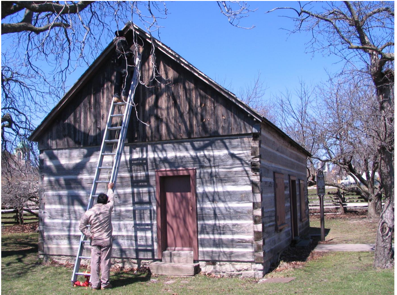
Above: Scadding Cabin repairs. Photo: David Raymont.
